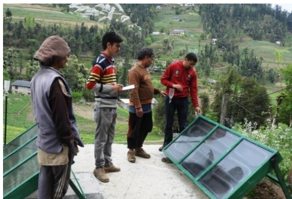
Installation of solar water heating systems in project area Mandi (HP)
