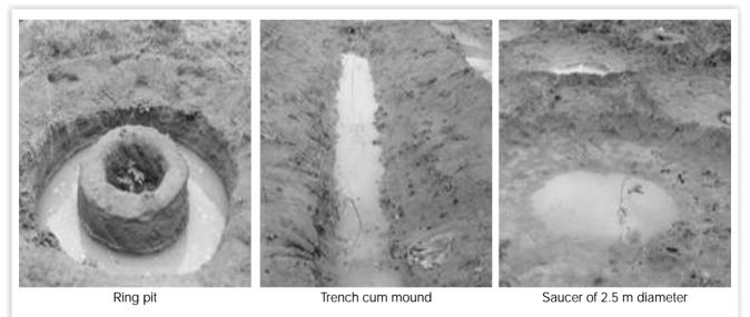
Fig 11.4. Different rain water harvesting structures
