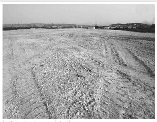
Fig 13. Top soil spreaded evenly on the backfilled quarry
