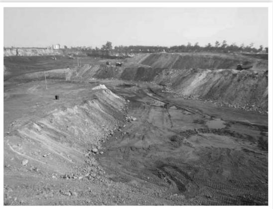
Fig 12. Backfilling of OB in exahusted pilot mine pit
